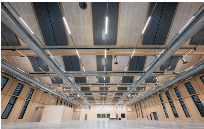
Top floor of the new Zephyr Hangar production building
